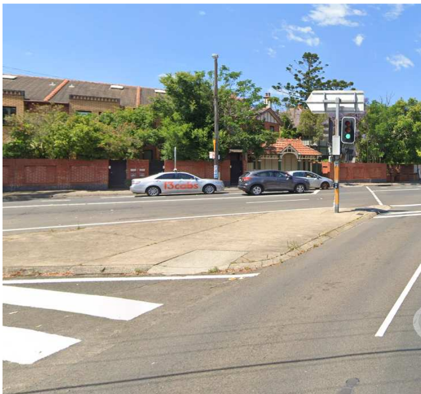
Figure 2.6: Pedestrian Crossing Frenchmans Road showing non complying kerb ramp.
