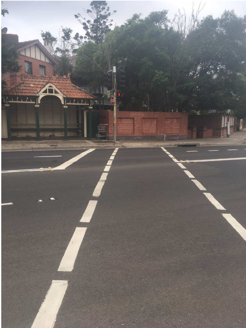
Figure 2.5: Pedestrian Crossing at Frenchmans Road and Randwick bound bus stop showing non complying kerb ramp.
